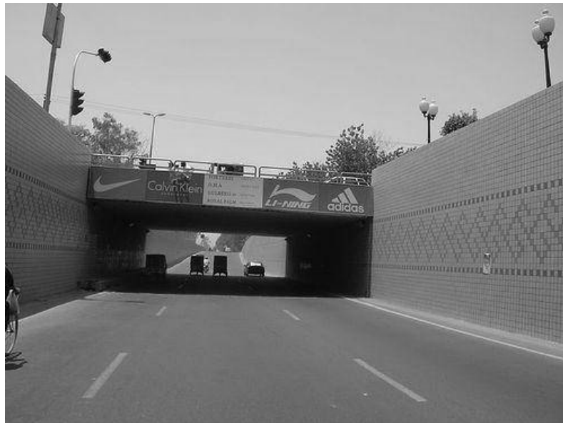
Figure 2.1.8 One of the Underpasses along Canal Bank Road
