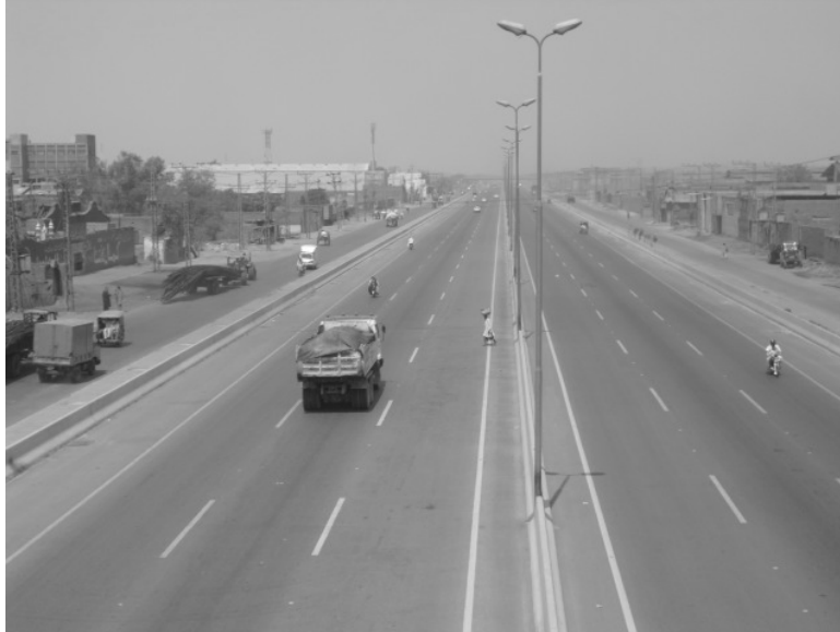
Figure 2.1.7 A Completed Section of Lahore Ring Road
