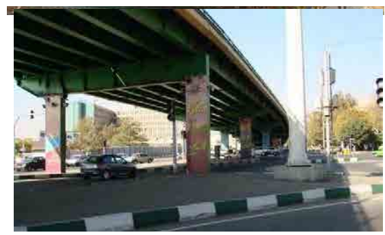
Fig6. Chamran-Jalal (Gisha) Bridge (orthotropic-Before 1990)
