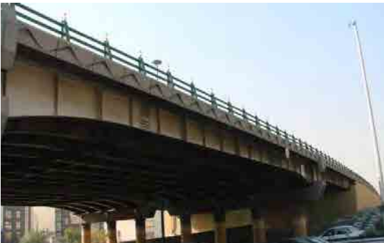
Fig1. Ashrafi Isfahani-Hakim Bridge (Steel-After 2000)
