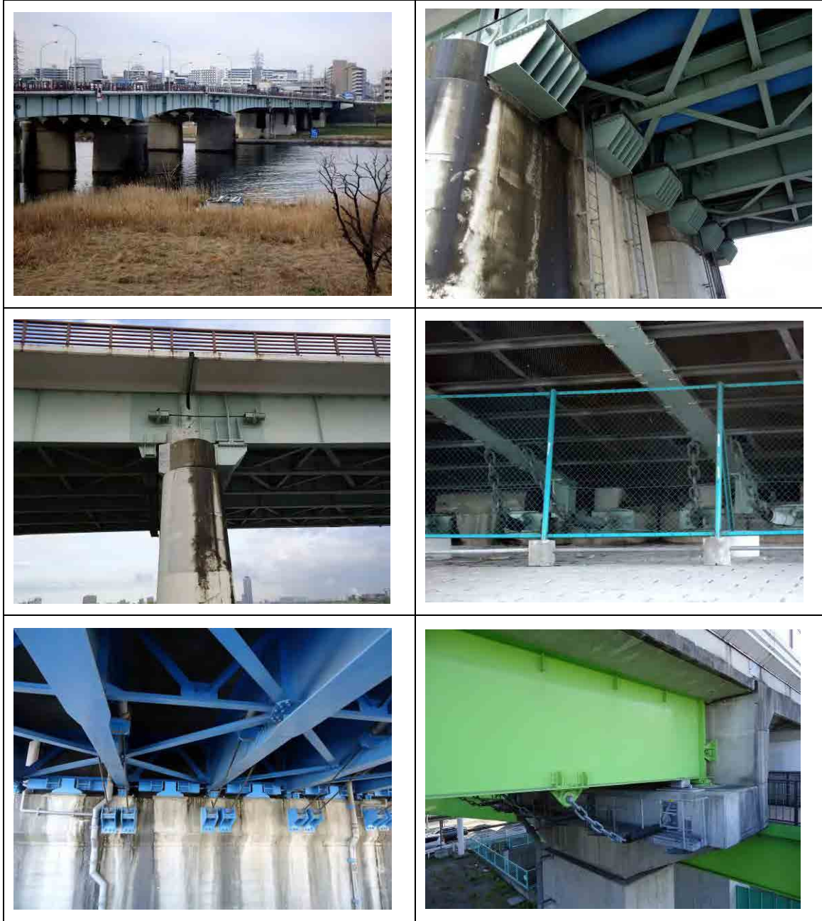
Photo 1 Seismic Retrofitting
