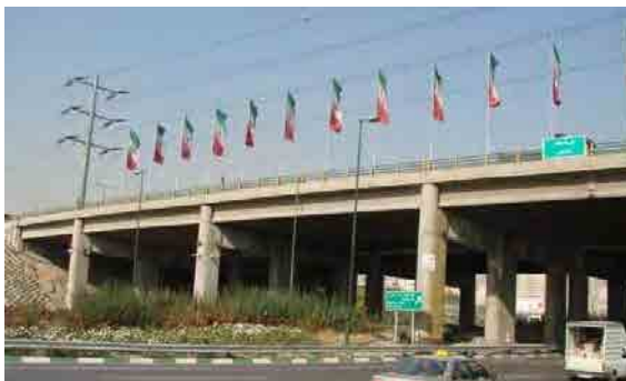
Fig5. Babaei-Imam Ali Bridge (concrete-after 2000)
