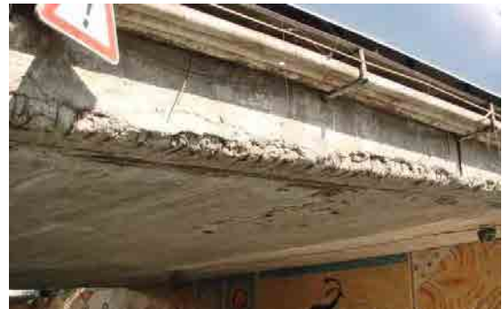
Fig4. Sadr-Bahar Bridge (Concrete-Before 2000)
