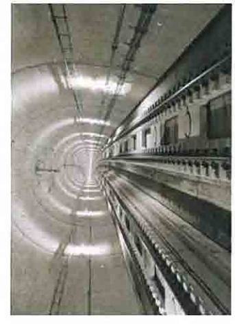
Tunnel (Kyushu Shinkansen)
