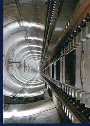
In a tunnel (Frame type slab track)
