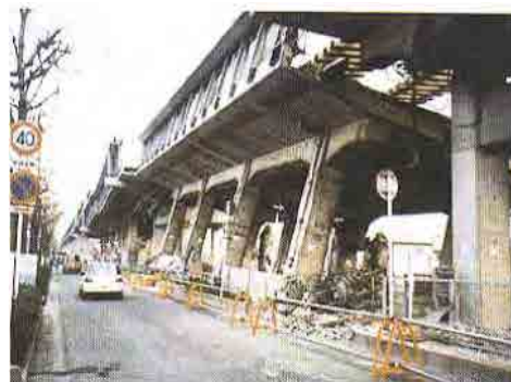
Figure 3-12 Damage to Sanyo Shinkansen Viaduct from Hanshin-Awaji Earthquake in 1995
