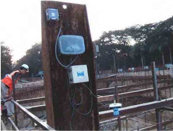
OSV Display (Blue & Yellow) for Ground Anchor Axial Force at Central College Station
