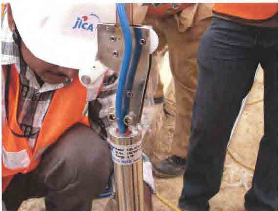
Installation of Inclinometer and OSV Display Equipment at Cricket Stadium Station
