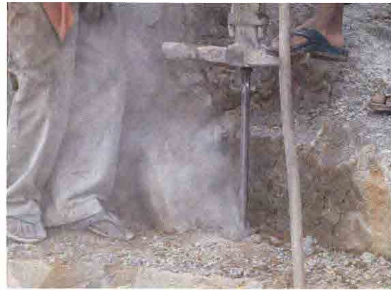
Dusty Condition under Rock Drilling Work
