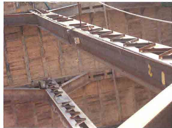
OSV Lighting for Axial Force of Strut monitored by Strain Gauge (Cricket Stadium St.)
