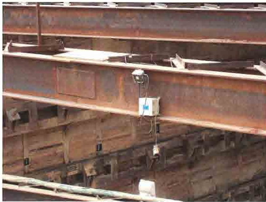
OSV Lighting for Axial Force of Strut monitored by Strain Gauge (Cricket Stadium St.)
