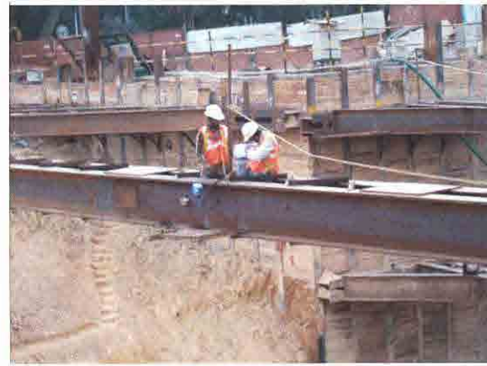
Installation of Strain Gauge for Strut Axial Force at Cricket Stadium Station
