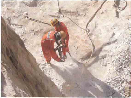
Dusty Condition under Rock Drilling Work
