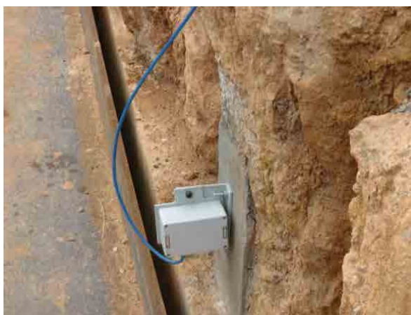
(a) Scan pile and a tilt meter
