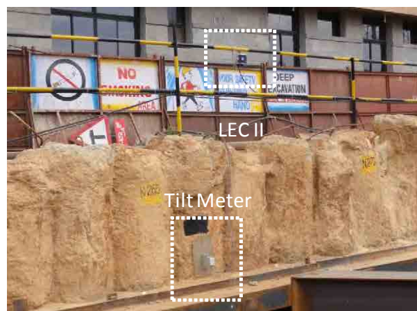
(b) Tilt Meter connected to LEC
