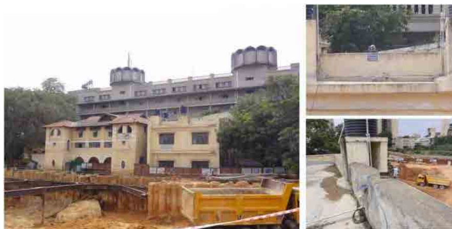
(b) BSNL building and a stand-alone LEC set up on its roof top
