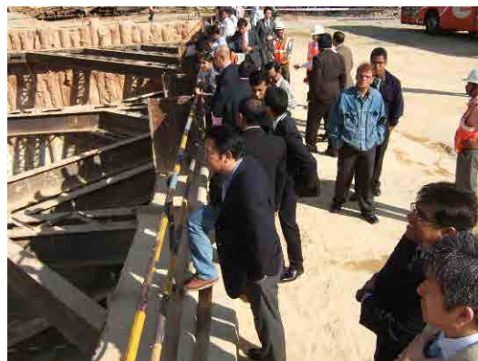
Figure 8.5 Picture of Workshop (Site Visit at Cricket Stadium Station)
