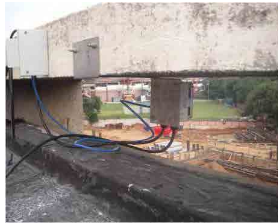
(c) LEC installation for workers
