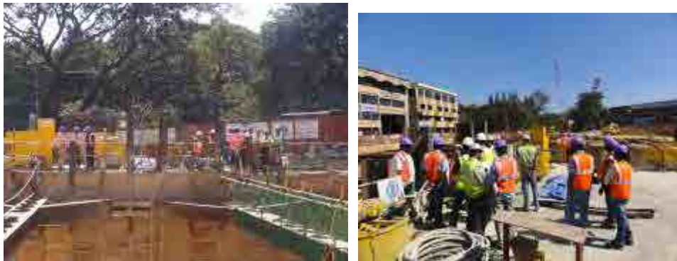
Figure 6.10 Permit to work inspection with BMRC/GC, Contractor and OSV team
