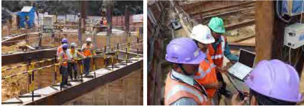
Figure 6.7 Daily site walk with BMRC/GC, the Contractor and JICA team
