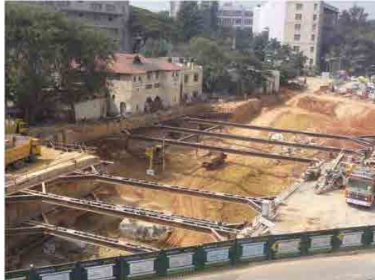
(a) BSNL building on the south-west corner of the excavation site
