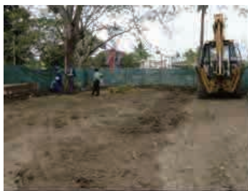
Compost site preparation at the Council depot
