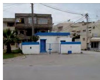
Photo: Station de pompage, Bizerte
