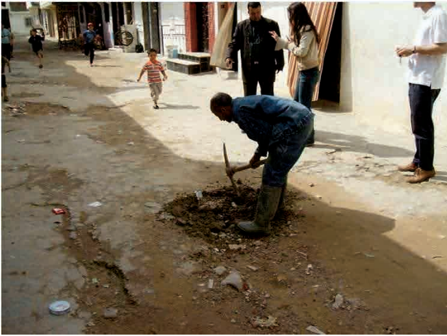
Buried manhole (Bizerte)
