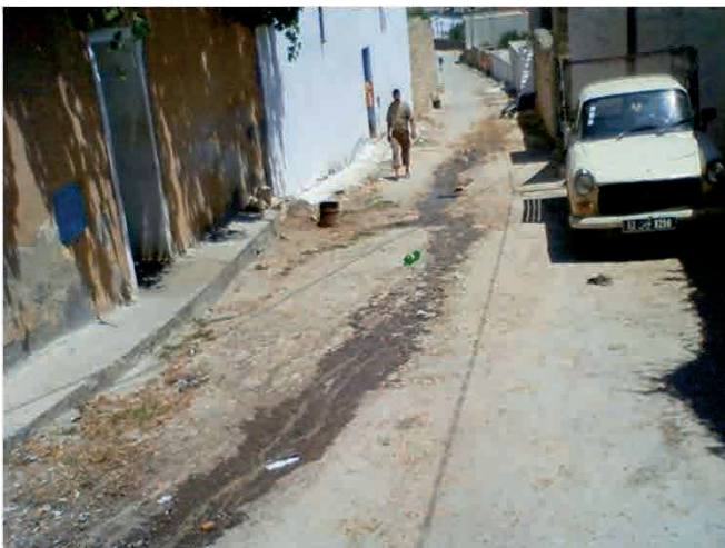
Leakage from choked manhole (Beja)
