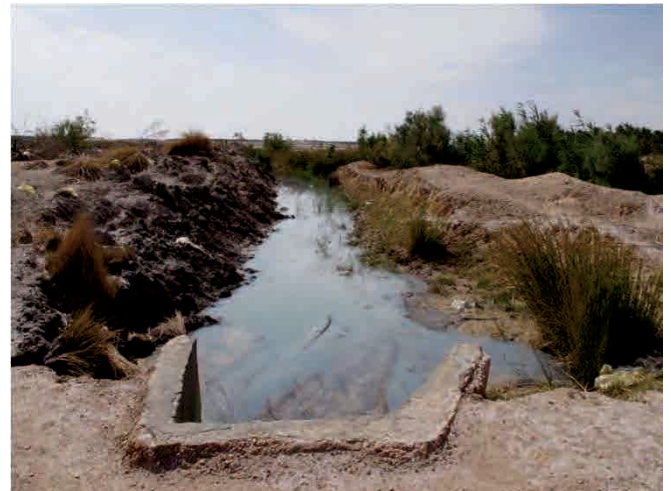
Discharge point to the chott (salt lake) without WwTP (Kebil)
