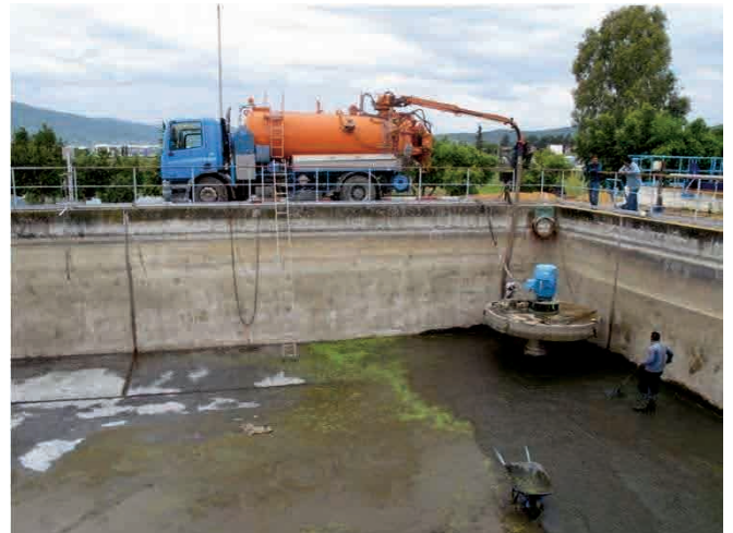
Aeration tank under periodic maintenance (WwTP Tabarka)
