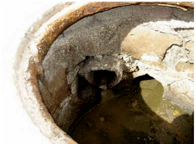
Degraded pipes of asbestos concrete (Beja)
