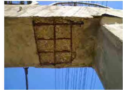
Feeder pillar's conditions
