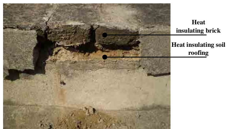
Photo 2: the surfaces of the roof
