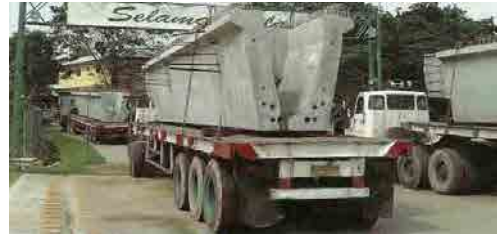
Photo-2: Transport of PC-U girder
