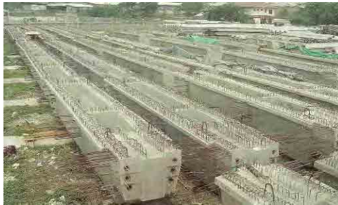
Photo-1: Precast PC-U girder
