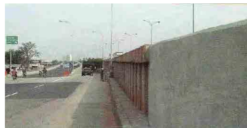
Photo-8: Completion of Driven Piles
