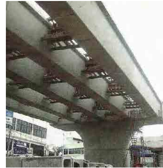
Photo-4: Form works of Diaphragm beam
