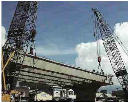
Photo-3: Erection of PC-U girder
