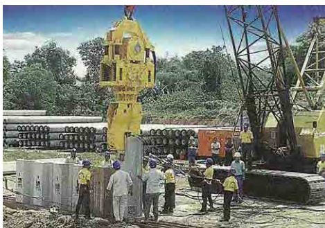
Photo-7: Driving PC Sheet Piles
