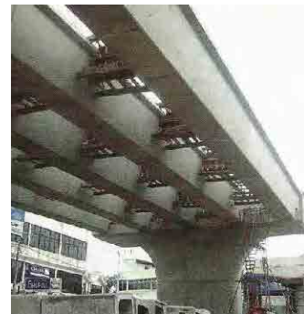
Photo-4: Form works of Diaphragm beam
