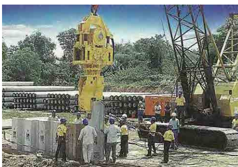
Photo-7: Driving PC Sheet Piles
