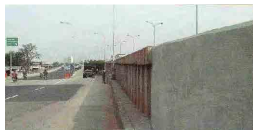
Photo-8: Completion of Driven Piles
