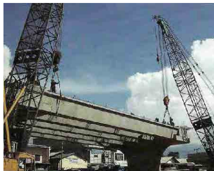
Photo-3: Erection of PC-U girder
