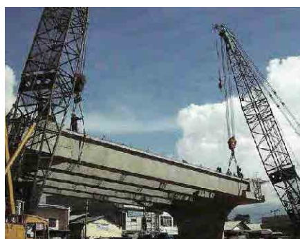
写真-3: PC-U 桁の架設
