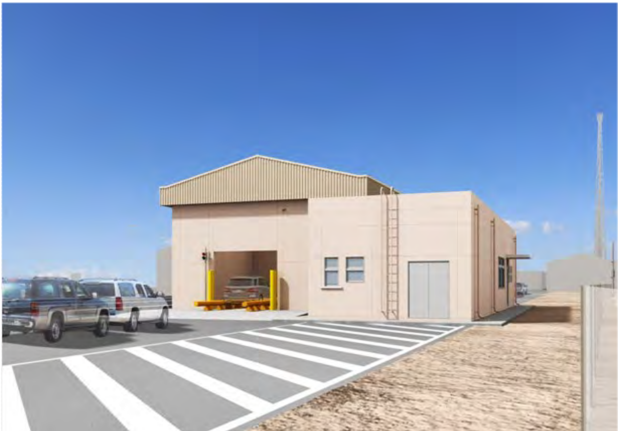
Passenger Car and Small Vehicle Inspection Building
