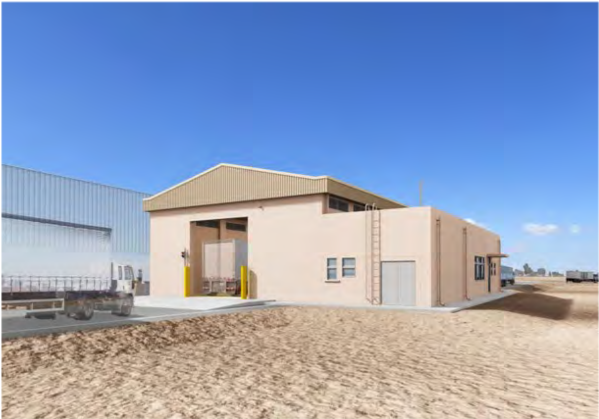
Cargo Inspection Building
