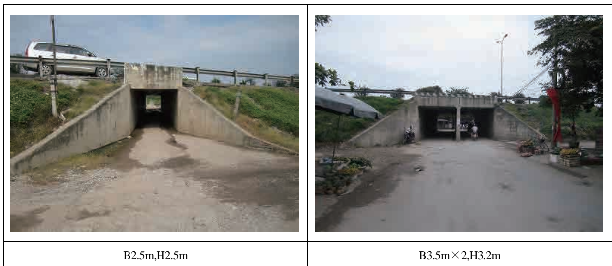
Figure 3.2.2-1 Existing Box culvert
