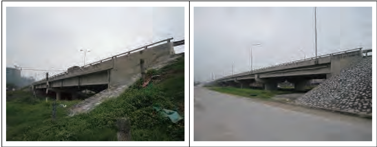
Figure 3.2.2-4 Van Dien Bridge
