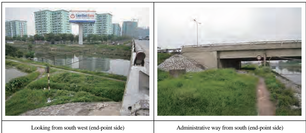
Figure 3.2.2-3 Van Dien Bridge
