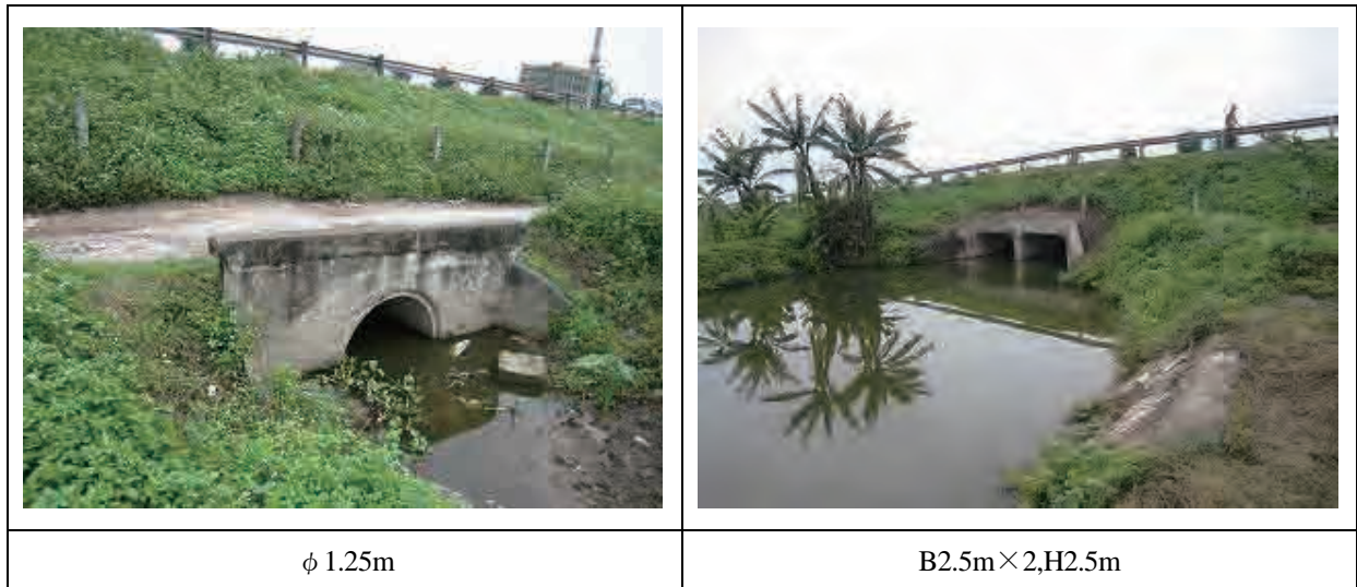
Figure 3.2.2-2 Existing Pipe culvert for drainage
