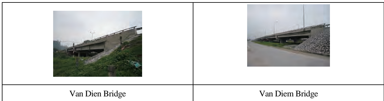
Figure 3.2-12 Existing Van Dien Bridge and Van Diem Bridge
