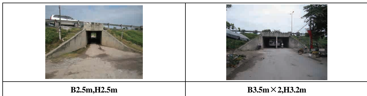
Figure 3.2-11 Existing Box culvert
