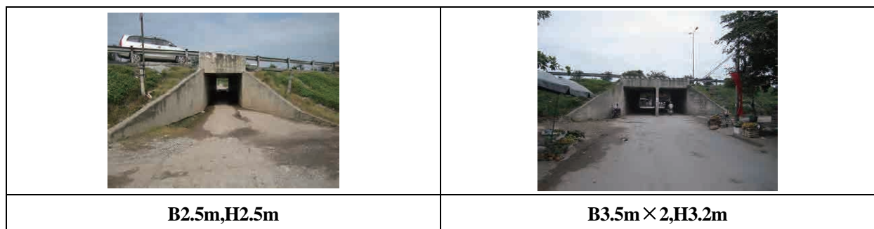
Figure 3.2-11 Existing Box culvert
