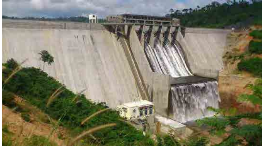
Figure 6 Main Dam and PH3 of Kamchay Hydropower
