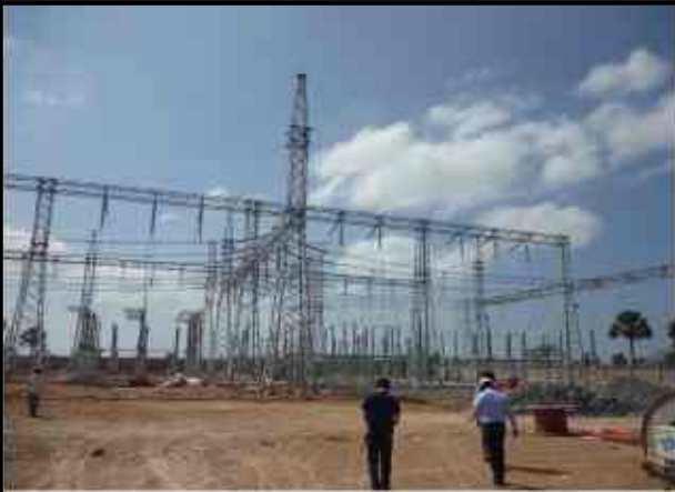
GS Kampot (Under Construction)
