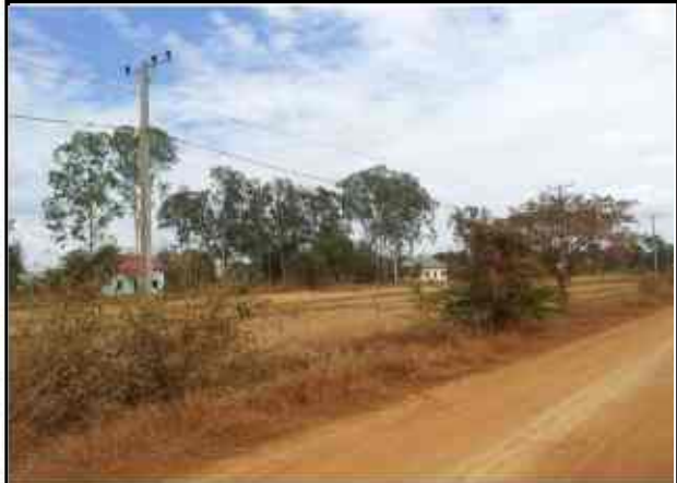
Distribution Line, Anlog Chrey Hydropower Project, Krang Ponley Irrigation Project
