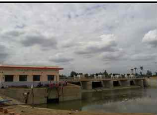
Powerhouse and Dam Spillway, Krapeu Truom Hydropower Project, Krang Ponley Irrigation Project
