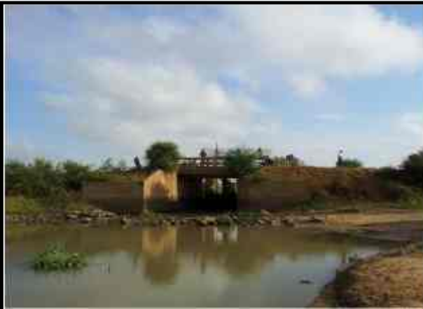
Draems Regulating Gate, , Kandul Stung Irrigation Project
