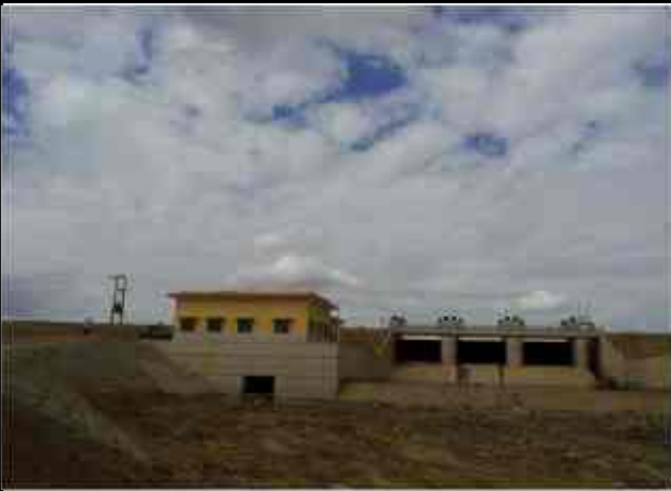
Powerhouse and Dam Spillway, Anlog Chrey Hydropower Project, Krang Ponley Irrigation Project
