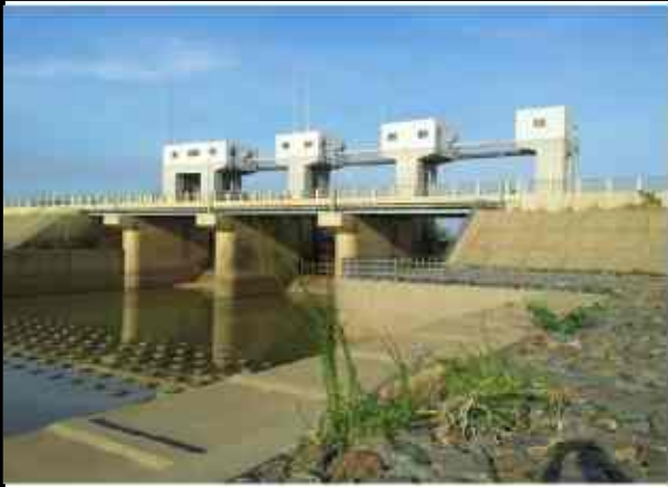
7th January Weir, Kandul Stung Irrigation Project
