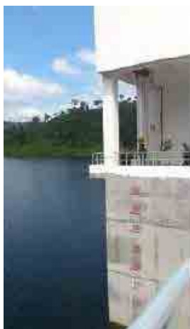
Figure 8 Water Level of Main Dam
