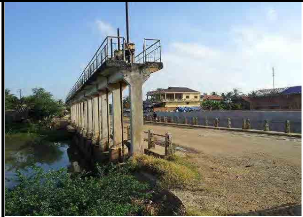
Tuk Tula Regulating Gate , Kandul Stung Irrigation Project
