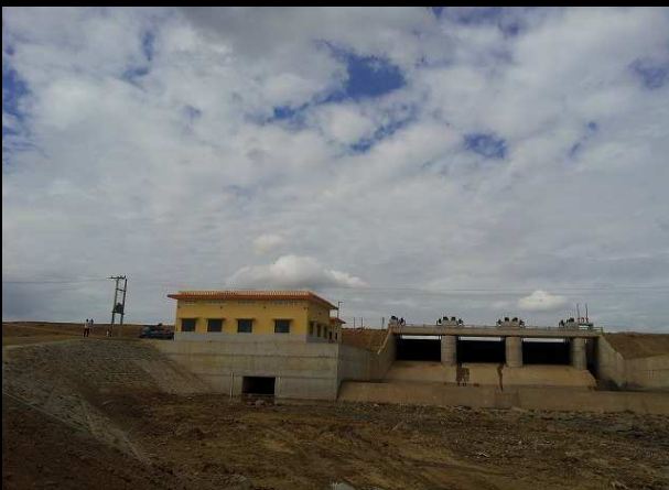
Powerhouse and Dam Spillway, Anlog Chrey Hydropower Project, Krang Ponley Irrigation Project
