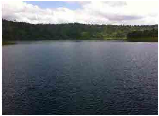
☒ 10 Reservoir of Main Dam
