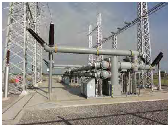
図 2 115kV Circuit (Gas Insulated Switch, GIS)
