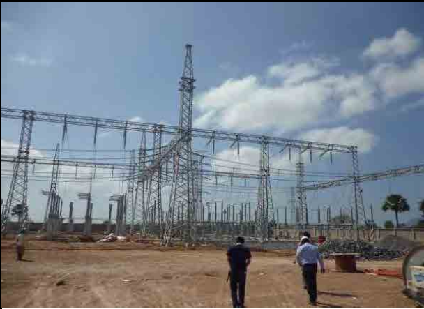
GS Kampot (Under Construction)
