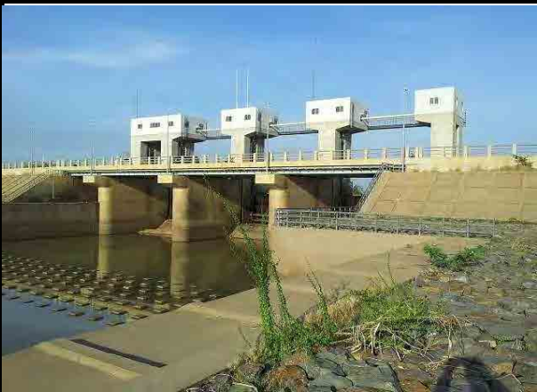
7th January Weir, Kandul Stung Irrigation Project
