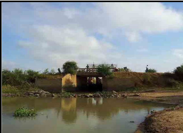
Draems Regulating Gate, , Kandul Stung Irrigation Project
