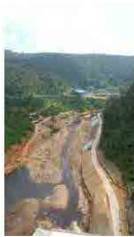
☒ 9 Downstream of Main Dam
