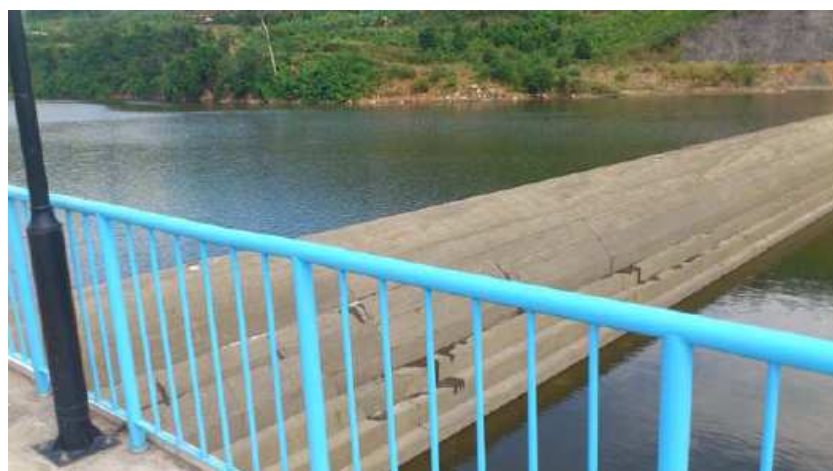
☒ 11 Re-regulating weir for PH1 (Weir for PH2)
