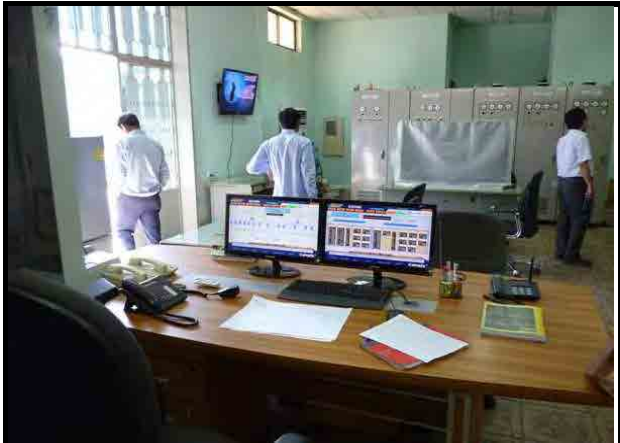
Control Room of GS3
