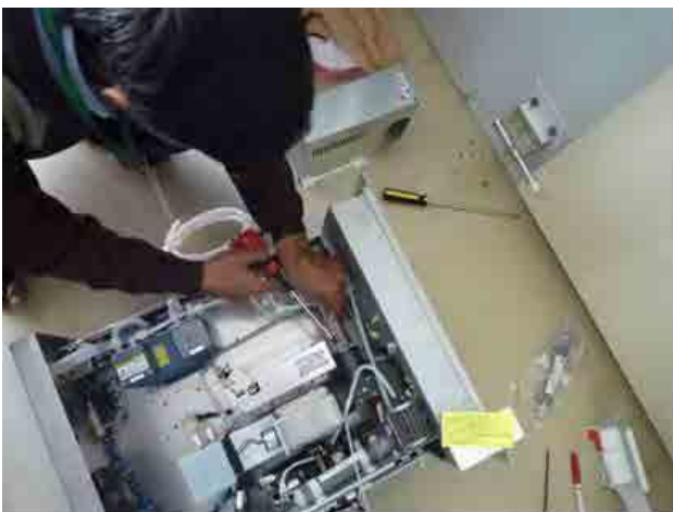
Photo-5 Repair Work on Air Monitoring Station, December 2009, Lahore
