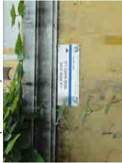
Installed Flood Mark Plates
