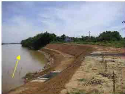
Overview from Upstream
