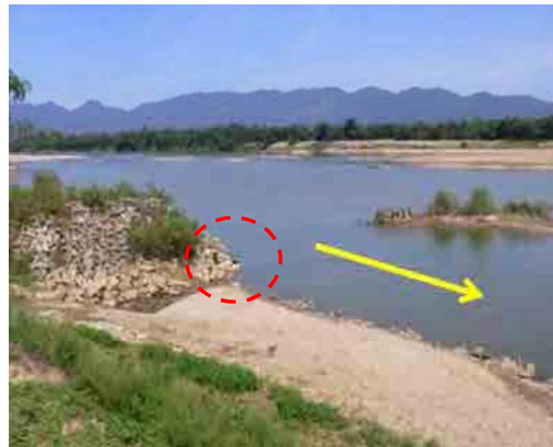
Current Condition of Stone Groin (as of Aug.2011)
