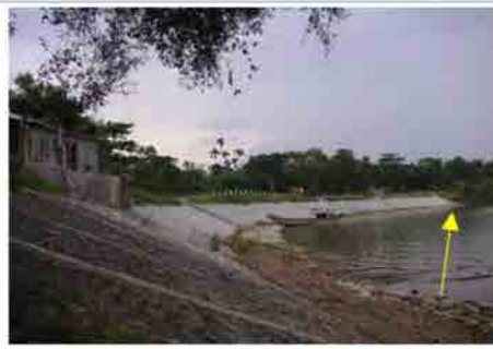
Completed Works (Upstream View)
