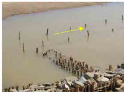
Bamboo Groin and Gabion
