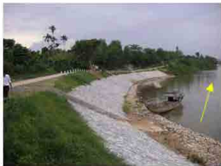
Completed Works (Upstream View)
