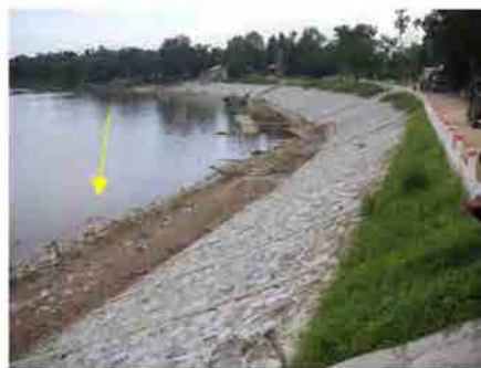
Completed Works (Downstream view)
