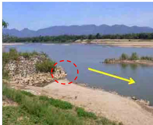
石積み水制の現状 (as of Aug.2011)
