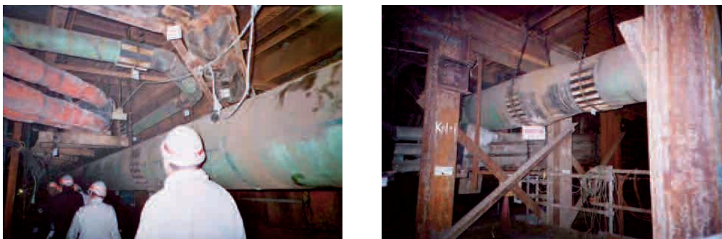
Figure 4.92 Temporary Hanging Method (Example)
