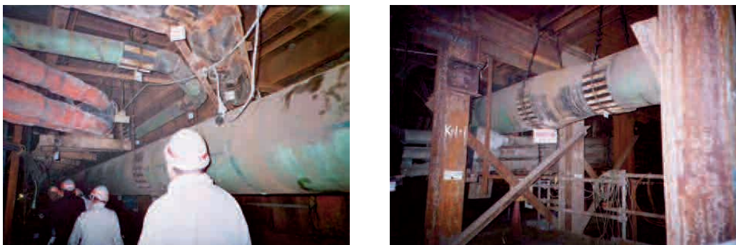
Figure 4.92 Temporary Hanging Method (Example)
