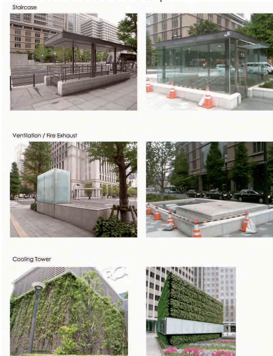
Figure 4.25 Incidents for Structures above Grade
