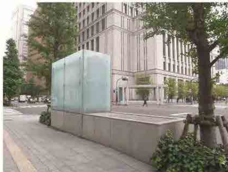
Ventilation / Fire Exhaust
