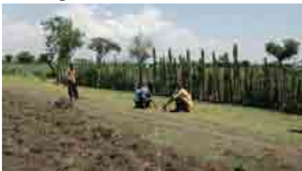
Oyne Umbure BH-3 (Electrode installation)
