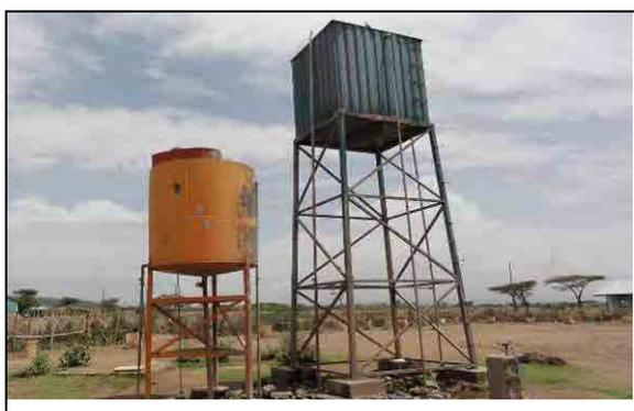
Mixing tank (left) and elevation tank
