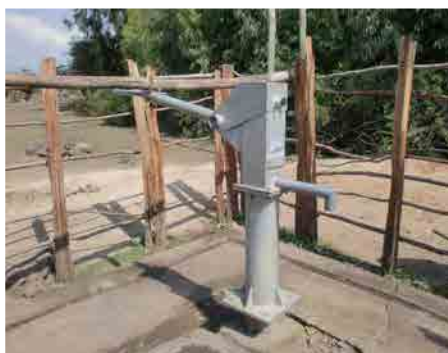
Hand pump system at Hams Gabaya
