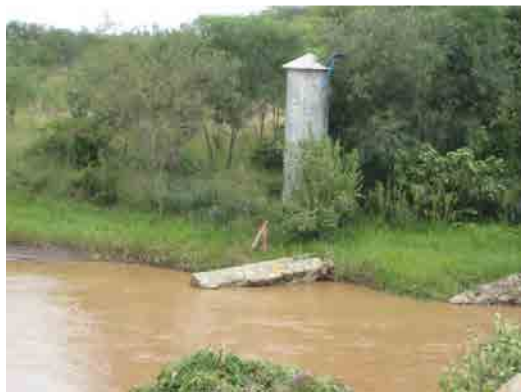
Figure 1.4: Gauging Station on Bilate River
