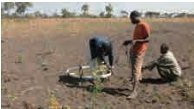
Induction coil installation (BH6)
