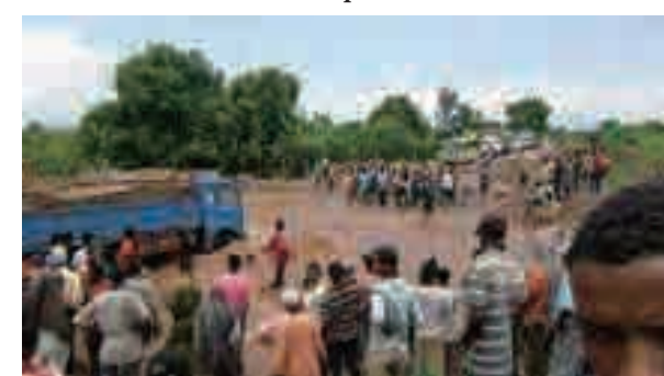
Sodo ~ Arbaminch road (Flooded culvert)
