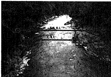
Photo - No.19 Kela Bridge
