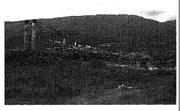
The piers are tilted because of scouring resulting from the insufficient width of the abutment footings and insufficient depth of embedding
