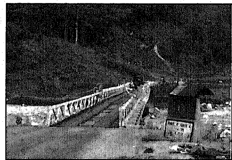
Photograph – An existing Bailey Bridge
