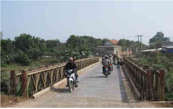
No.52 EA SUOP BRIDGE
