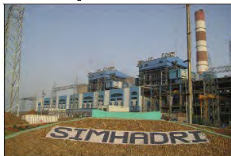
Simhadri Thermal Power Station
