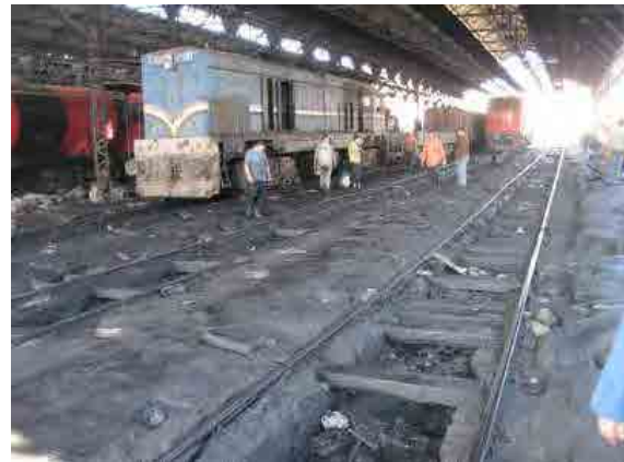
Figure 2.5.9 Inspection Track of Workshop
