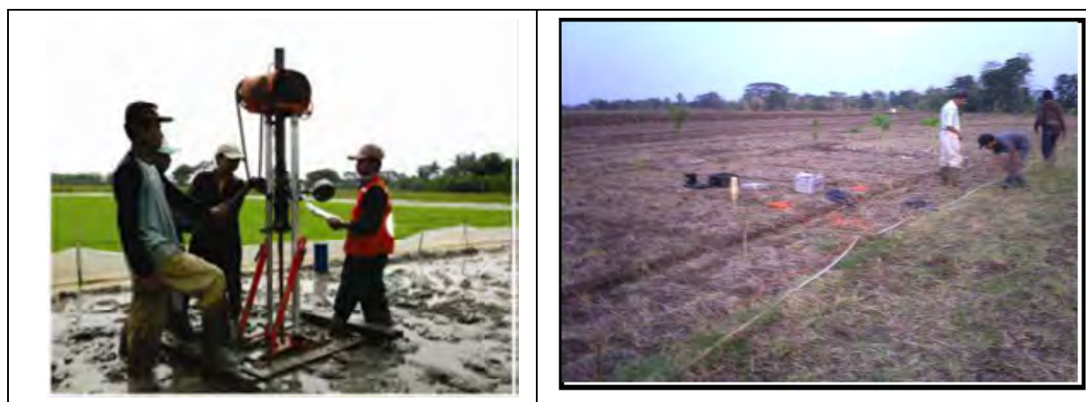
Photo 4.1 Site Survey Scene of DCPT(Left) and Seismic Refraction Survey(Right)
