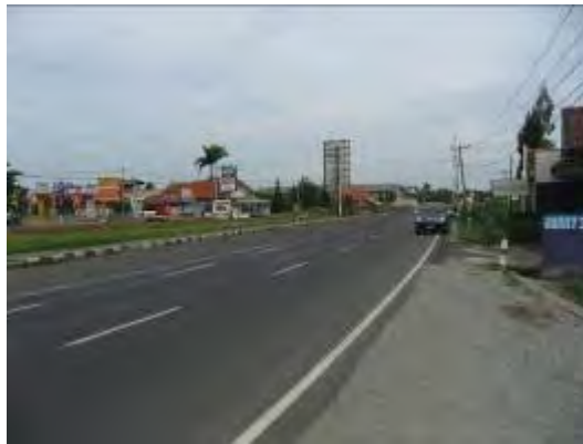
National road crossing between T.197 and T.198
