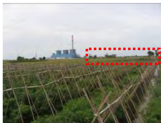
Indramayu P/S site
