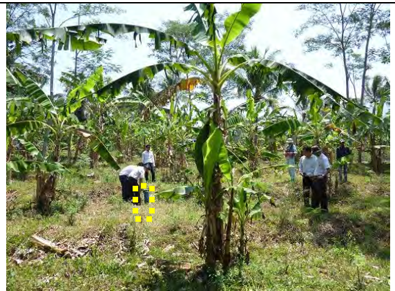
T.004 tower site (heavy angle)
