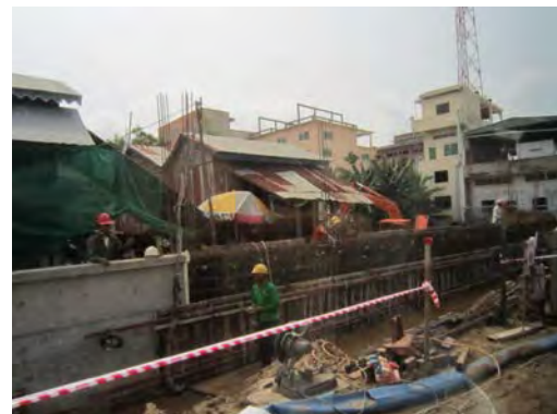
Work in the vicinity of private house
