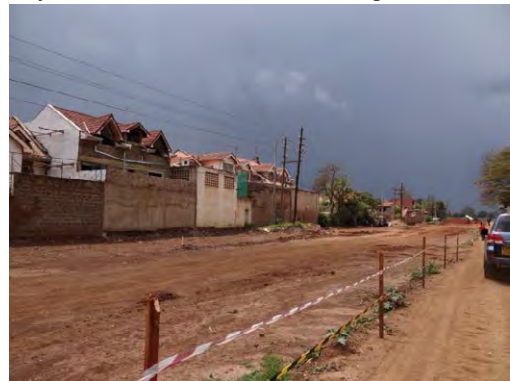
Project for the Construction of Nairobi Western Ring Roads ②
