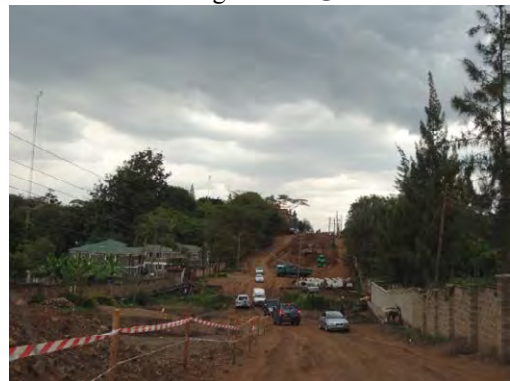
Project for the Construction of Nairobi Western Ring Roads ④
