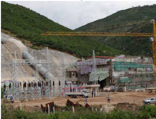
Sondu-Miriu Hydropower Project Sang'ro Power Plant Project ③
