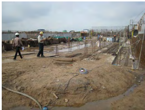
Niroth Water Supply Project ③
