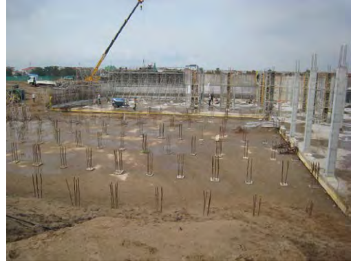
Niroth Water Supply Project ②
