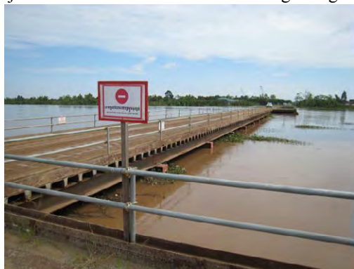
Project for Construction of Neak Loeng Bridge ③
