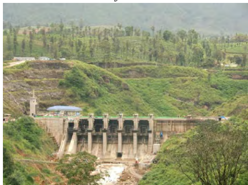
Upper Kotmale Hydro Power Project ②
