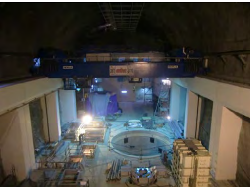
Upper Kotmale Hydro Power Project ③
