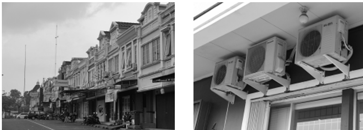
Figure 2.5.4-10 Ruko's Facade and Example of AC Installation
