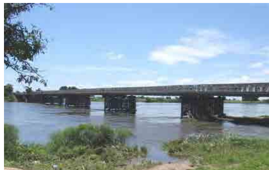
Photo-3 Existing Juba Bridge as seen from Downstream
