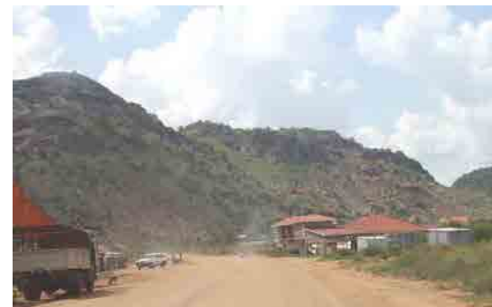
Photo-6 Existing Unpaved Section of R-1/C-3
