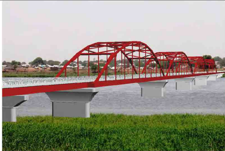
View from east bank
