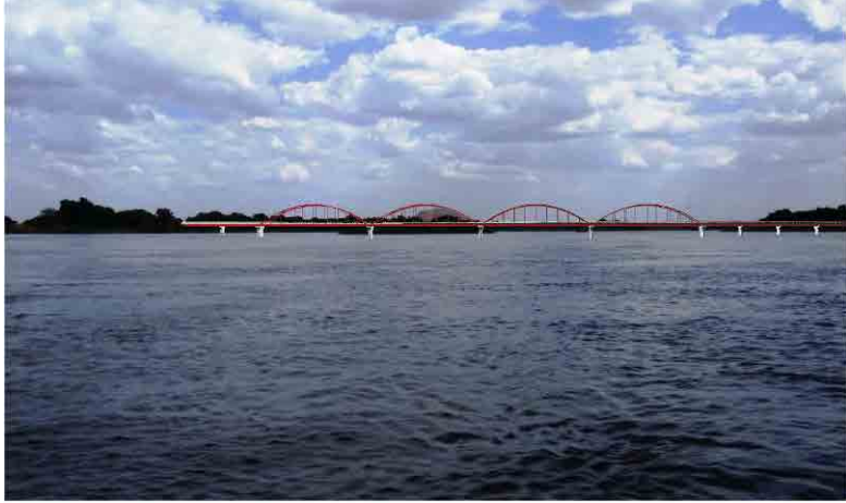
View of the bridge from downstream of Nile River
