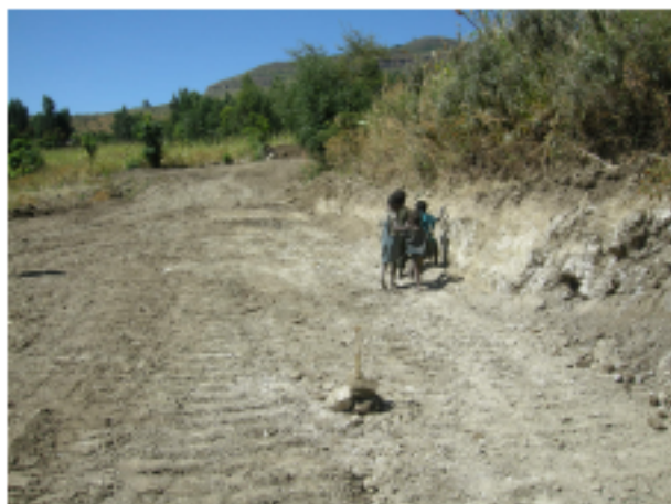
Construction of access road for drilling point B28-12 (sorghum field)
