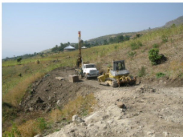
Construction of access road for drilling point B28-33 (sorghum field)
