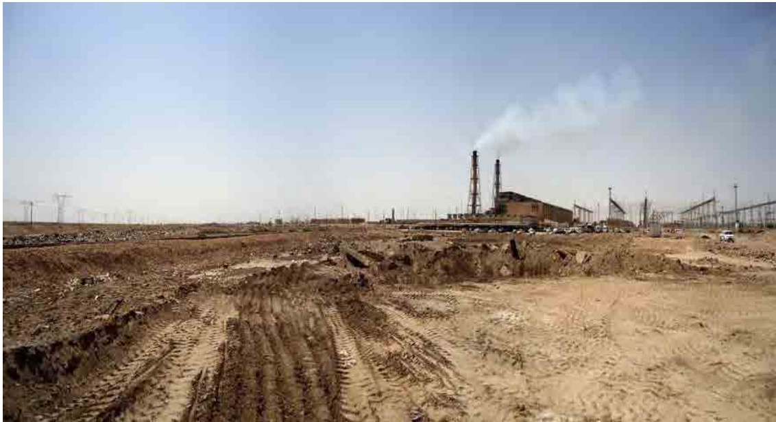
Photo 5-4-1 Photograph of the site (provided by MOE)
