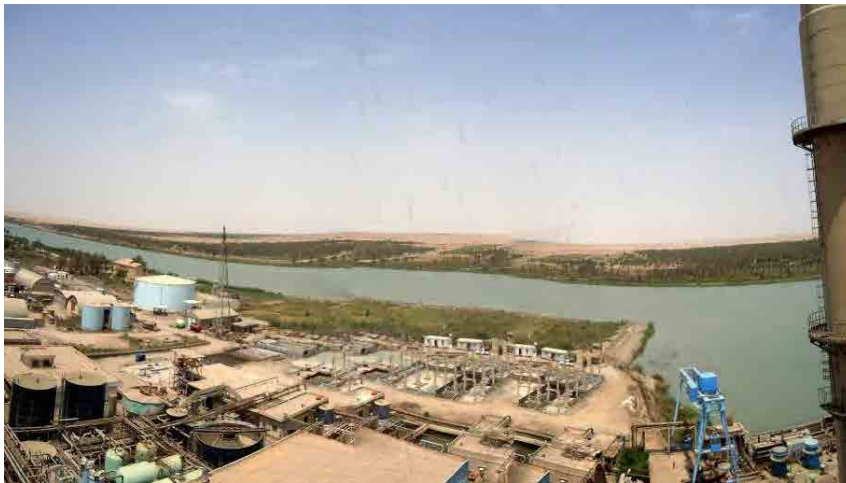
Photo 3-2-2 Hartha II Project Site (upstream of the existing Hartha PS)
