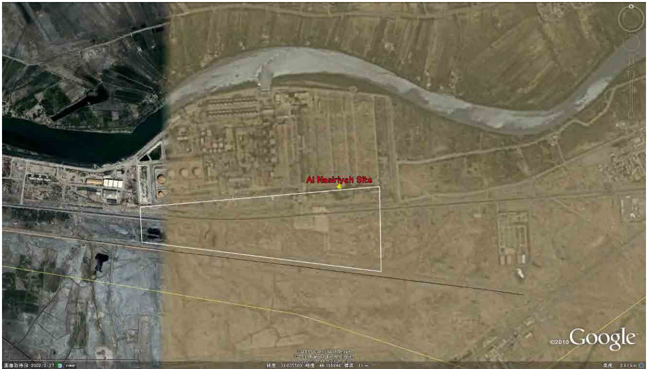
Figure 3-2-3 Nasiryah II project site (by Google Earth)
