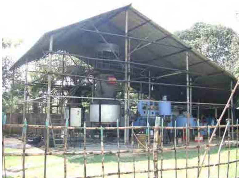
Figure 10.3.6.4 Biomass gasified generation plant
