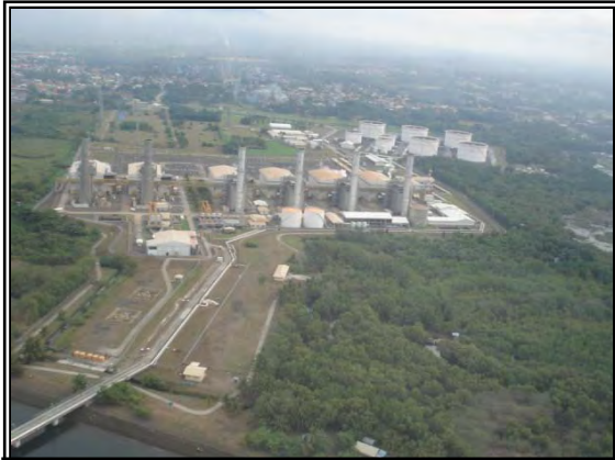
IRIJAN natural gas fired power plant Existing Malampaya OGP Facility
