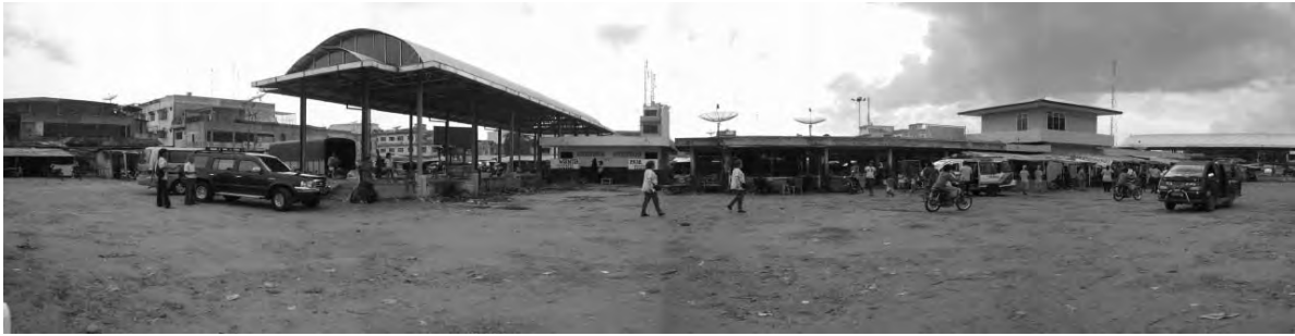
■ Overview image of the market: Loading space (left side), and other market buildings
