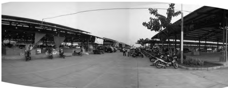
■ Overview of internal road and market buildings
