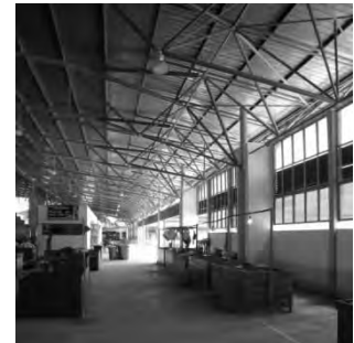
■ Roof truss (space frame)
