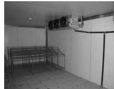
■ Internal condition of cold storage
