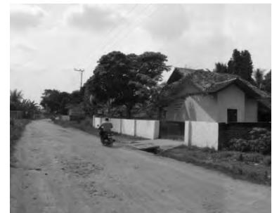
■ Private junior high school which is facing to access road
