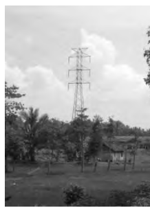
■ High-voltage line and tower in the site
