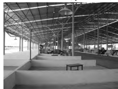
■ Market building with booth partitions and internal truck road
