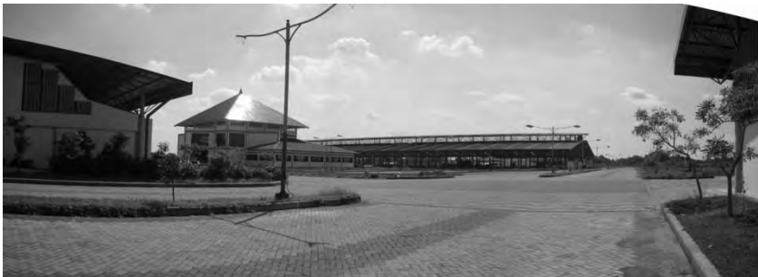
■ Overview of internal road and market buildings
